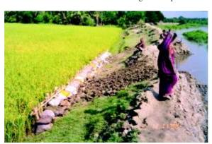
Photo 4.2: Embankment on the verge of collapse
